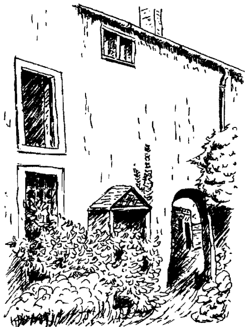
Fig. 74. Brewery Lane passing through the corner of the Spread Eagle inn, shortly before demolition.
